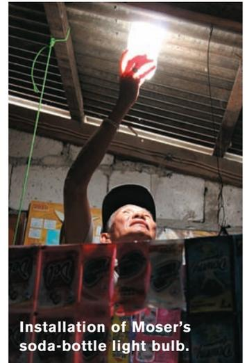
Installation of Moser’s soda-bottle light bulb.
