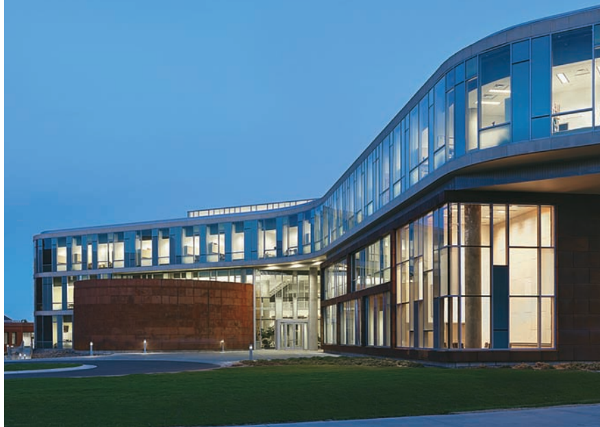
The new building for the Labovitz School of Business and Economics at the University of Minnesota, Duluth, reflected its commitment to its undergraduate program and took its name from the primary donor to the new facility. Photo copyright © James Steinkamp, Steinkamp Photography
