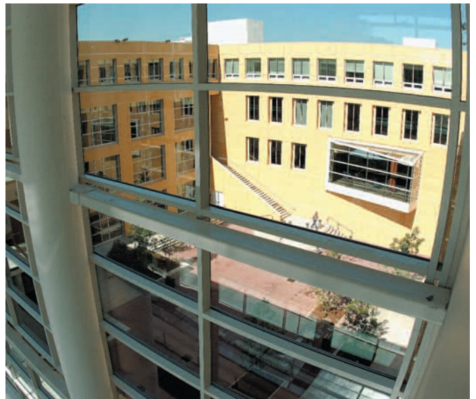
Georgia Tech's new building for its College of Management earned a silver LEED rating in 2003 for efficient and energy-conscious design.
